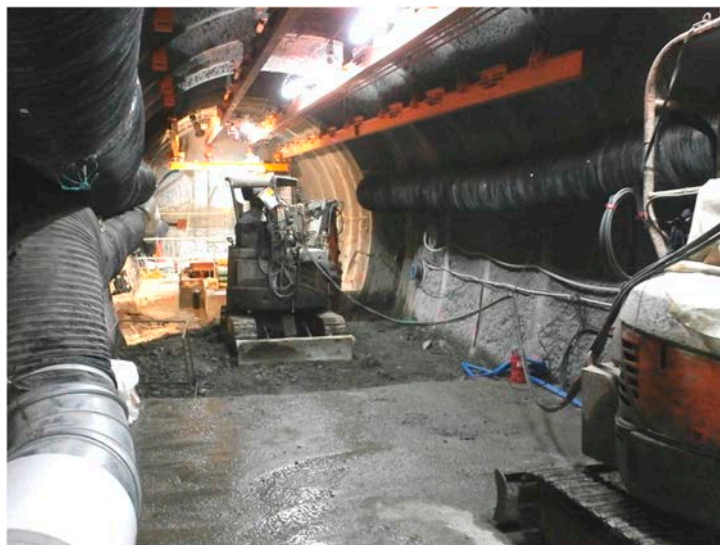
Photo 6 Excavation cutout of lower part for plug
