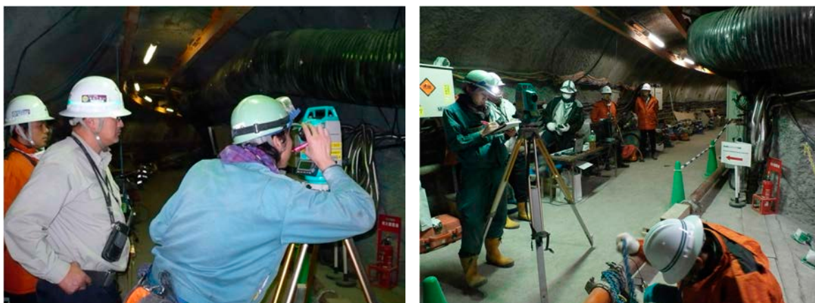
Photo 107 Measuring displacement of formwork
