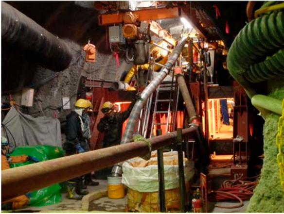
(a) Pumping concrete (outside of formwork)
