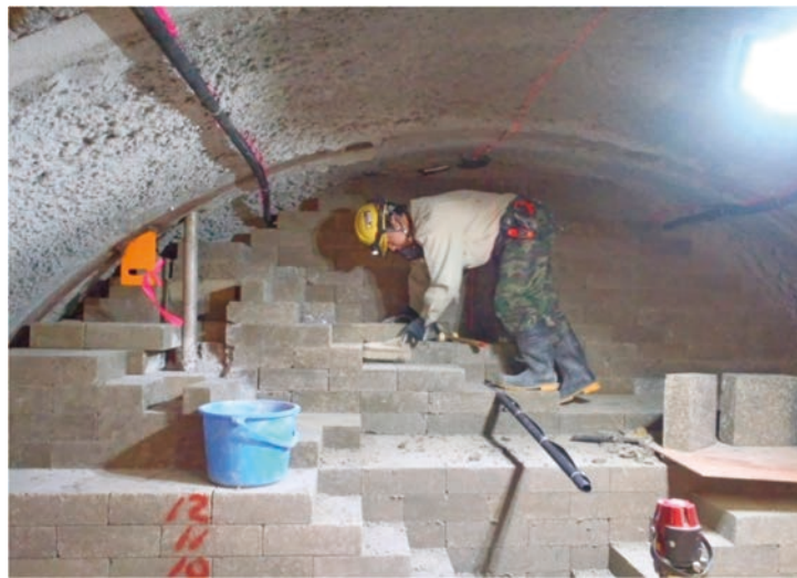
Photo 79 Setting situation (until 5th section, 25 layers)
