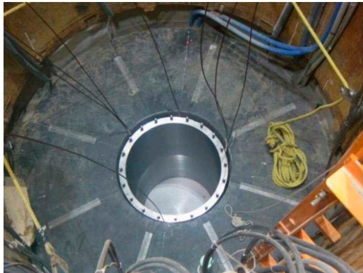
Photo 53 Setting simulated OP into the center of buffer material blocks
