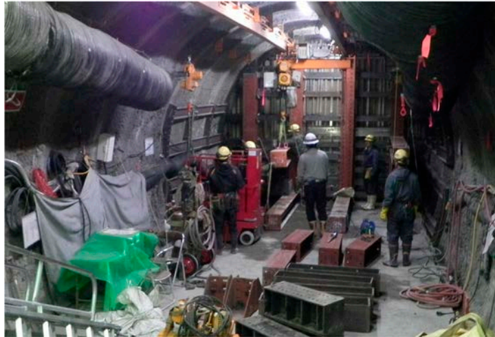
(a) Removal of bracing
