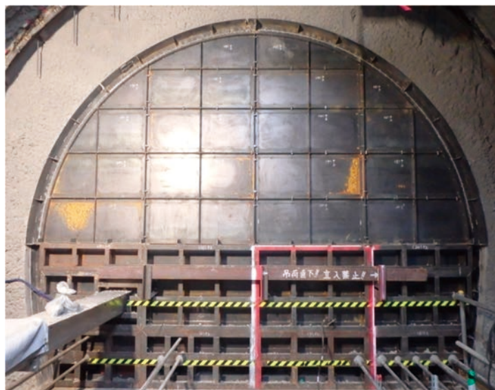
Photo 82 Setting a partition wall
