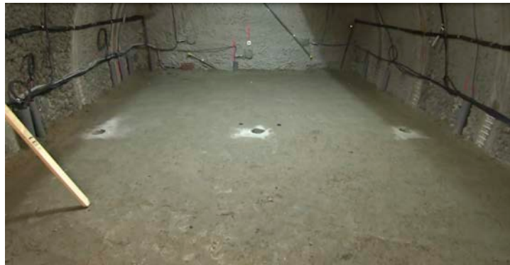
Photo 71 After compaction (Layer No.30)
