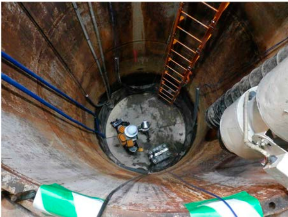
(a) Measurement at bottom of the pit
