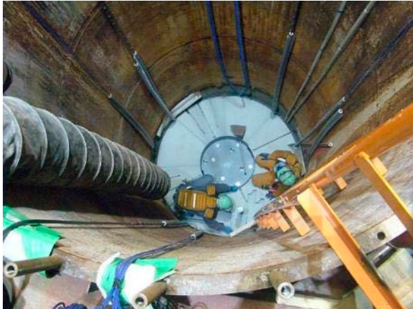
Photo 45 Working situation in test pit
