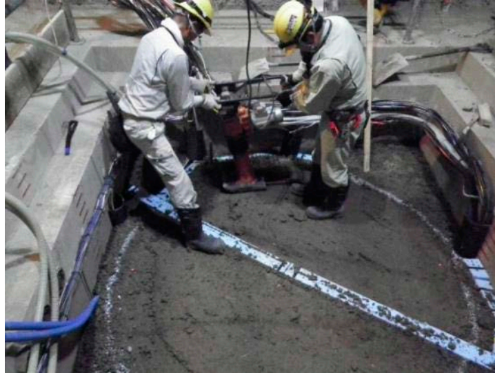
Photo 61 Compaction using rammer (Layer No.1)
