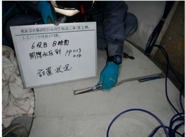
Photo 46 Setting a piezometer to chase of buffer material block
