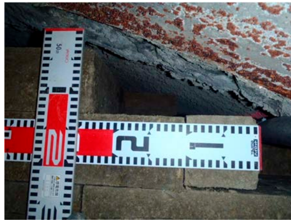
(c) Section 15, Layer 24 (right side) Photo 86 Measuring clearance
