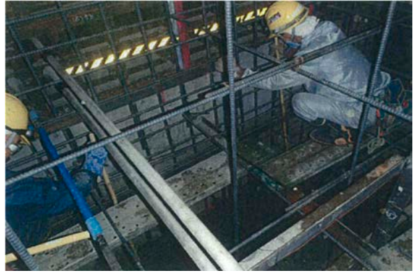
(b) Inside of formwork
