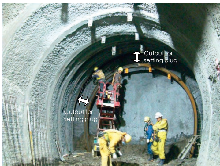
Photo 3 Widening for concrete-type plug
