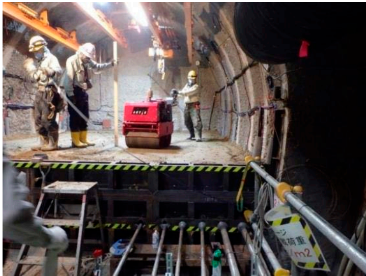
Photo 67 Compaction by hand guide roller
