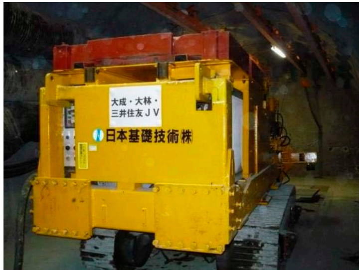
Photo 9 Setup drilling machine at Niche No.4 (rear view)
