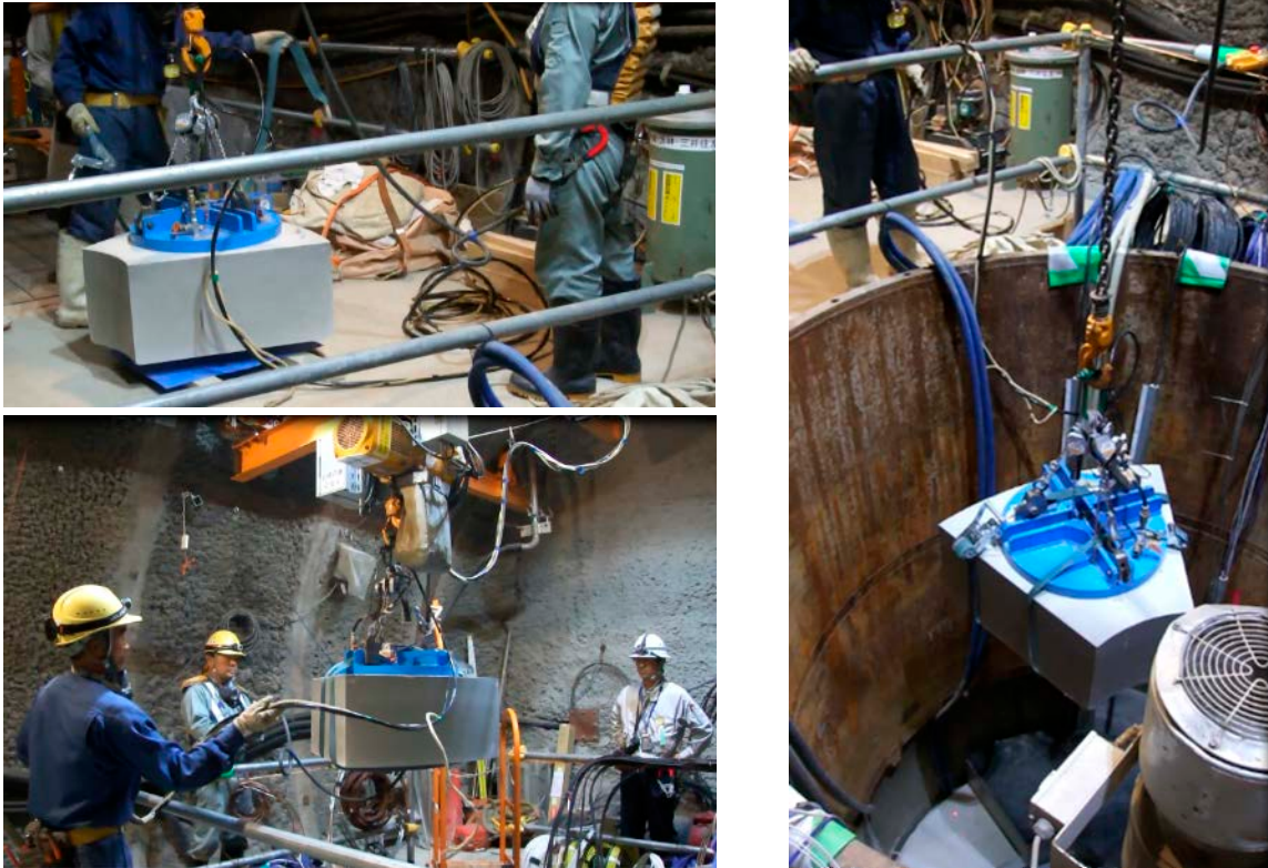
Photo 40 Setting buffer material block using vacuum grasp system
