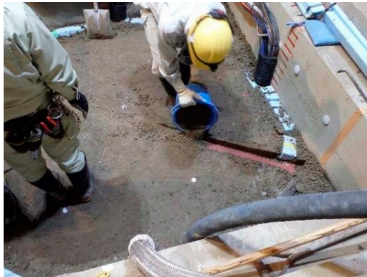
Photo 62 Infilling a chase with backfilling material
