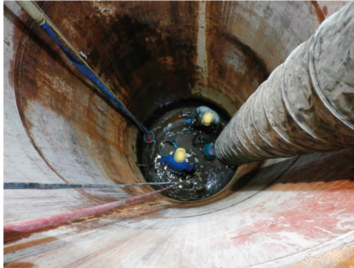
Photo 13 Completion of test pit excavation
