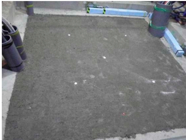
Photo 64 After Compaction of backfilling material (Layer No.12)
