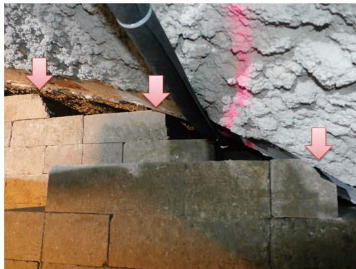
Photo 78 Setting blocks cutting of edge
