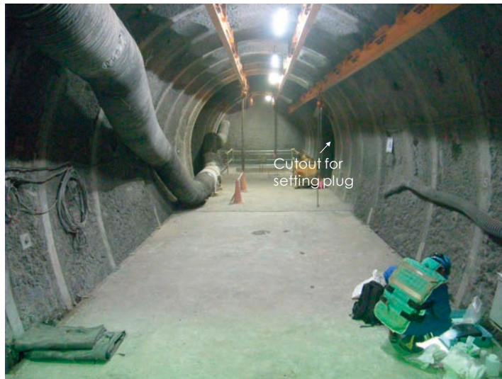
Photo 5 Niche No.4 after casting roadbed concrete
