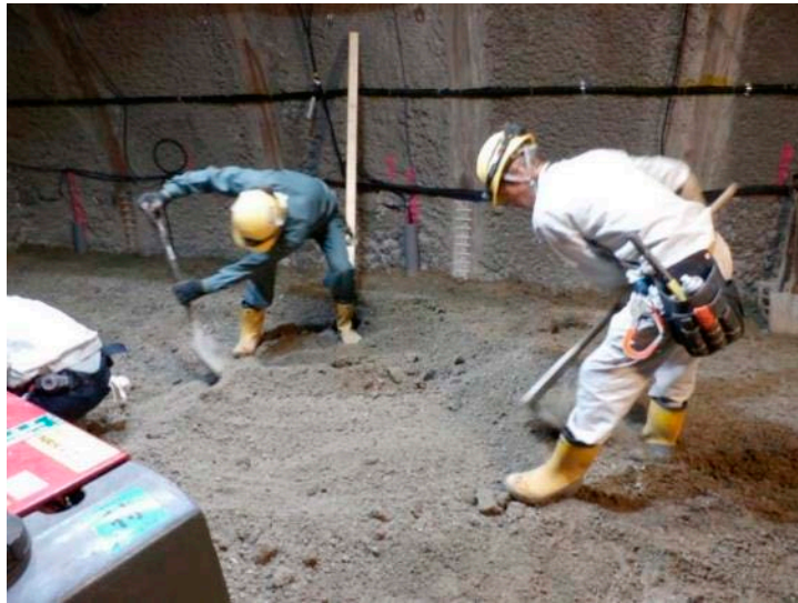
Photo 66 Instration and leveling backfilling material
