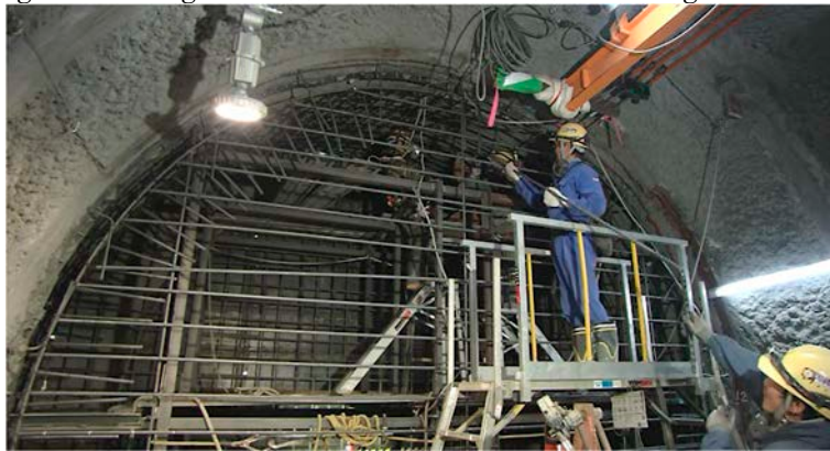
(c) Setting reinforcing steel (3)
