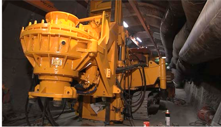
Photo 8 Setup drilling machine at Niche No.4 (front view)
