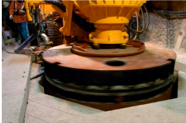
Photo 10 Drilling test pit by casing
