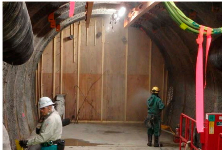
(c) Removal of formwork (2)
