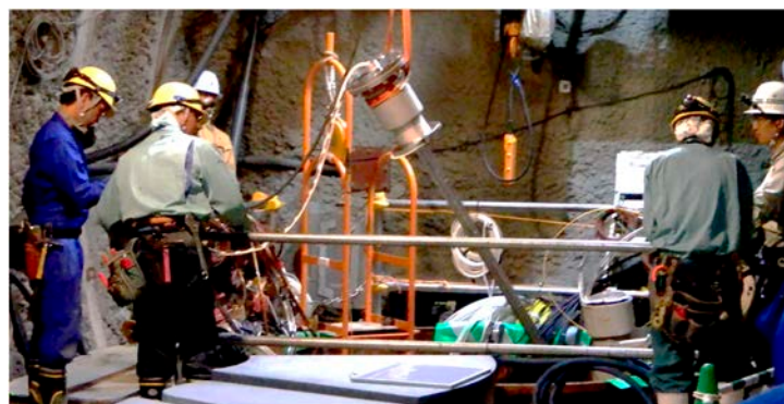
Photo 57 Move heater into test pit
