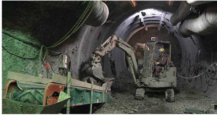
Photo 2 Taking out excavated rocks by conveyor
