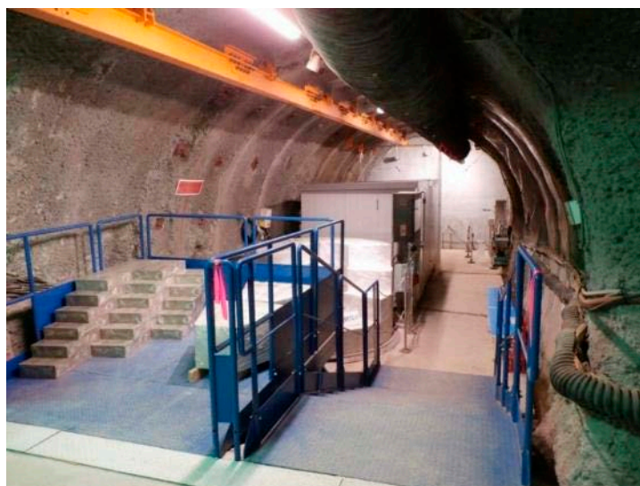
Photo 124 Full view of Niche No.4
