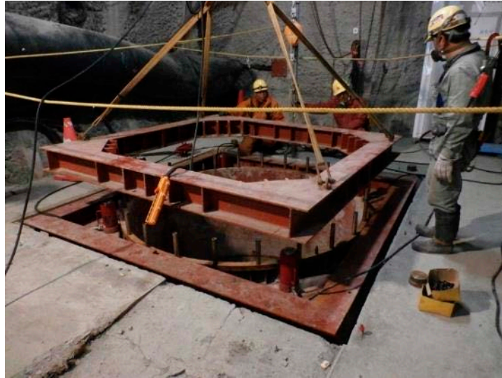
Photo 15 Steel frame for casing jack-up
