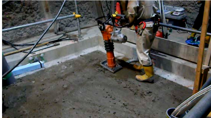
Photo 63 Compaction layer No.12 by rammer
