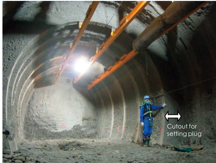
Photo 4 Niche No.4 before casting roadbed concrete
