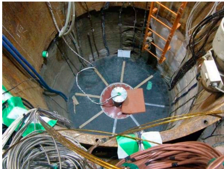
Photo 59 Completed setting simulated OP
