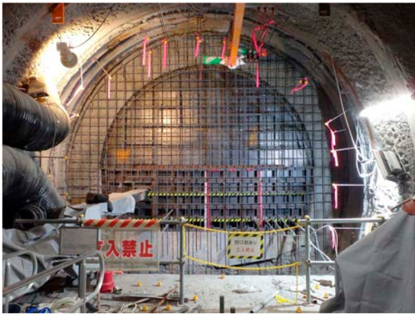
(a) Setting reinforcing steel (1)
