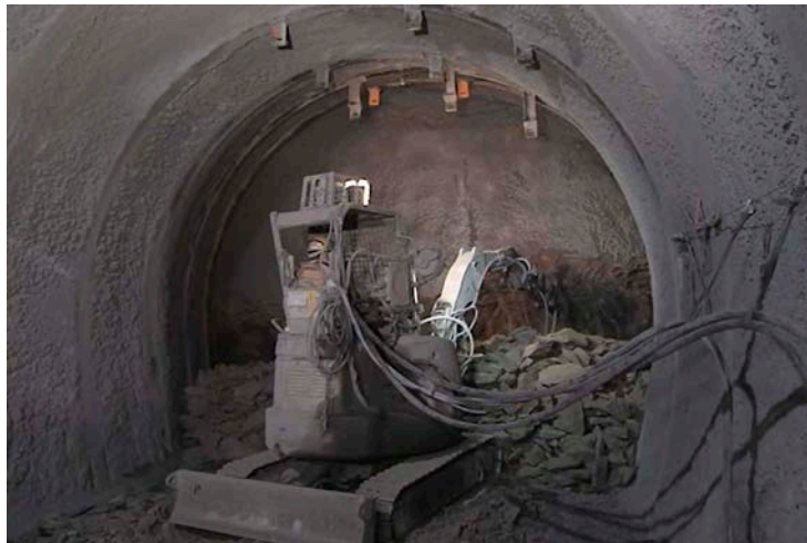
Photo 1 Excavation of Niche No.4 using hydraulic breaker
