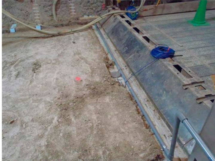
Photo 68 Wall for backfilling material guards
