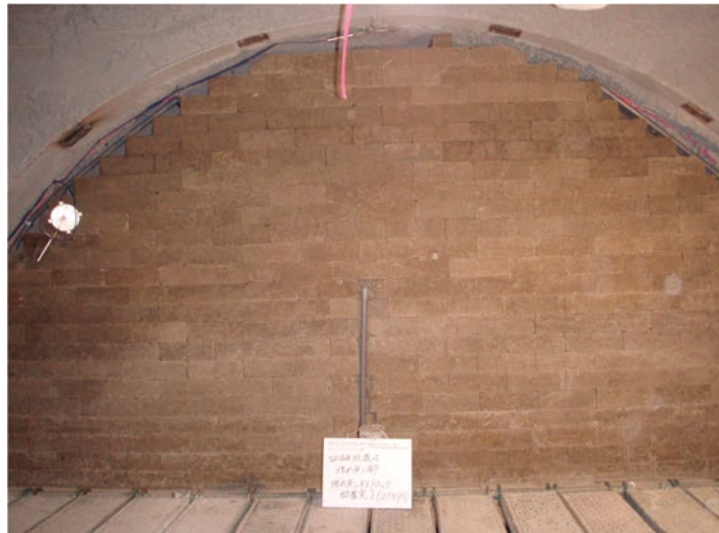
Photo 81 Completion setting blocks
