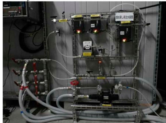
(c) For the backfilling material
