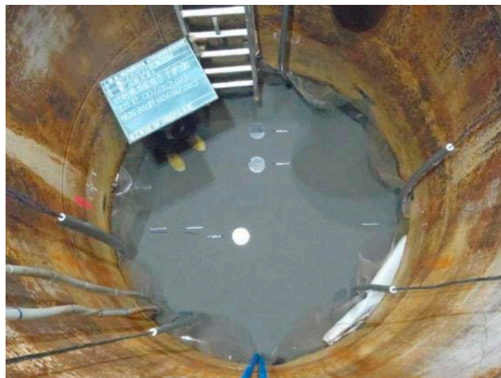
Photo 44 Setting sensors at the bottom of test pit
