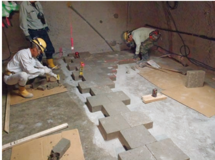
Photo 77 1st layer blocks setting
