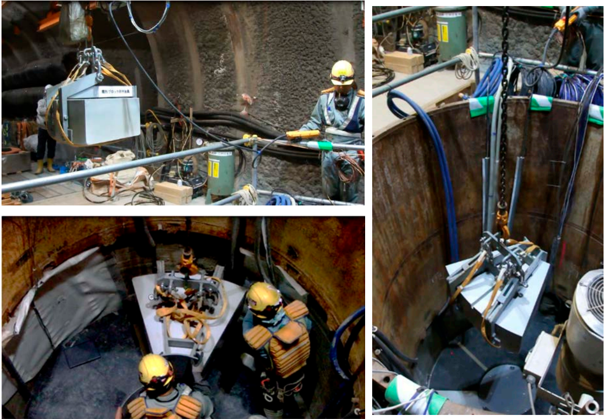
Photo 43 Setting buffer material block into test pit using mechanical grasp system
