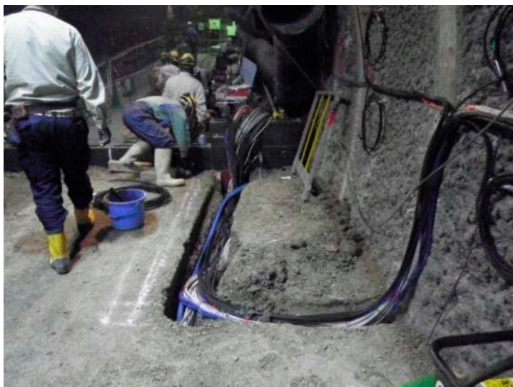
Photo 70 Laying sensor cables
