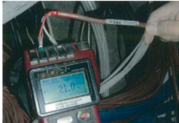
(b) After backfilling (TEOP005)
