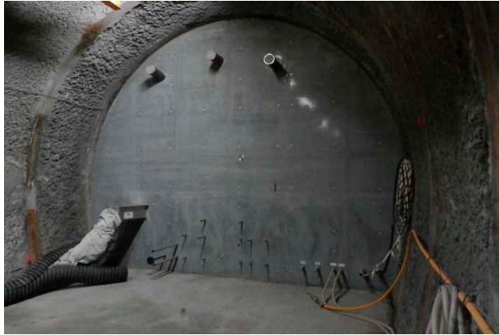
Photo 109 Completion of demolding
