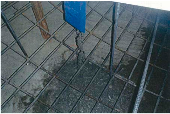
(c) Casting concrete using hose
