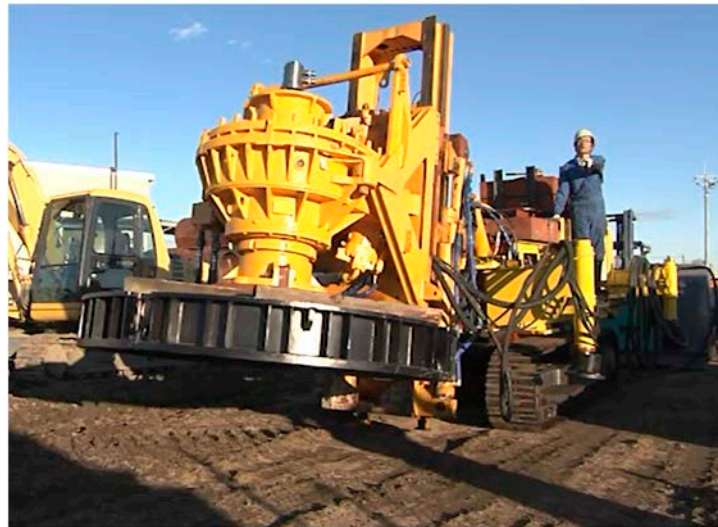
Photo 7 Drilling machine for large diameter
