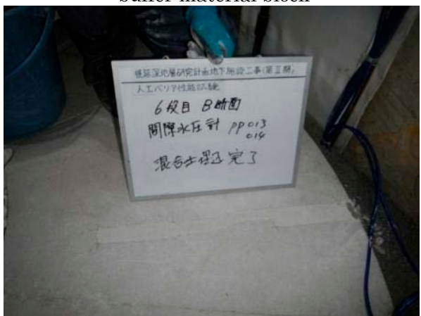
Photo 48 After infilling a chase
