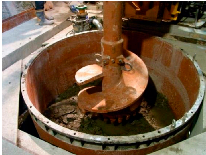
Photo 11 Drilling test pit by auger
