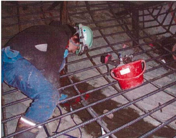
(a) Setting pressure cell
