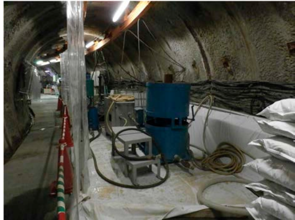
(b) Grout mixer
