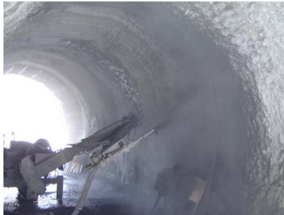
Figure 2.2.6-2 HFSC shotcreting test using mock up tunnel
